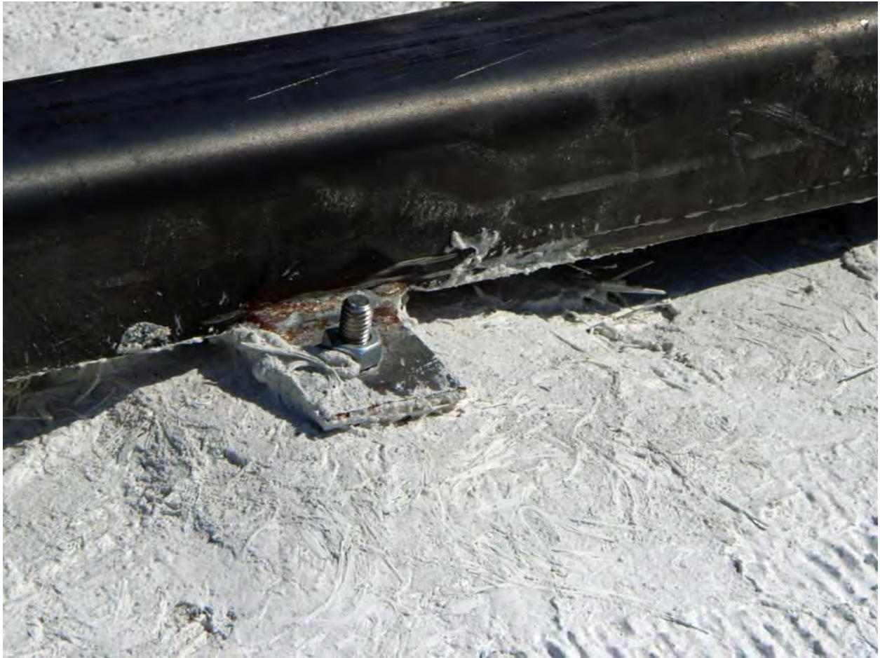
This slide shows the local thickening of the GRC necessary for the bigHead method of construction.
